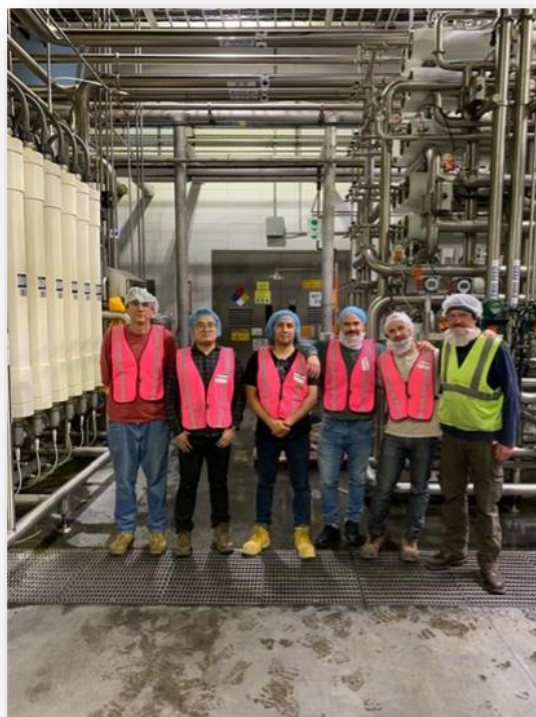
The Team onsite after the successful startup and installation of the Flow Reversal System.
