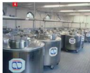
4: Vacuum insulated line for cryobiological storage
