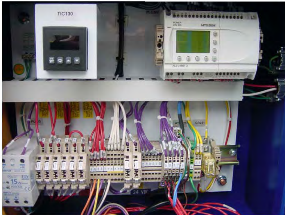
Figure 9 - Trifecta X-Series Control Box (open)
