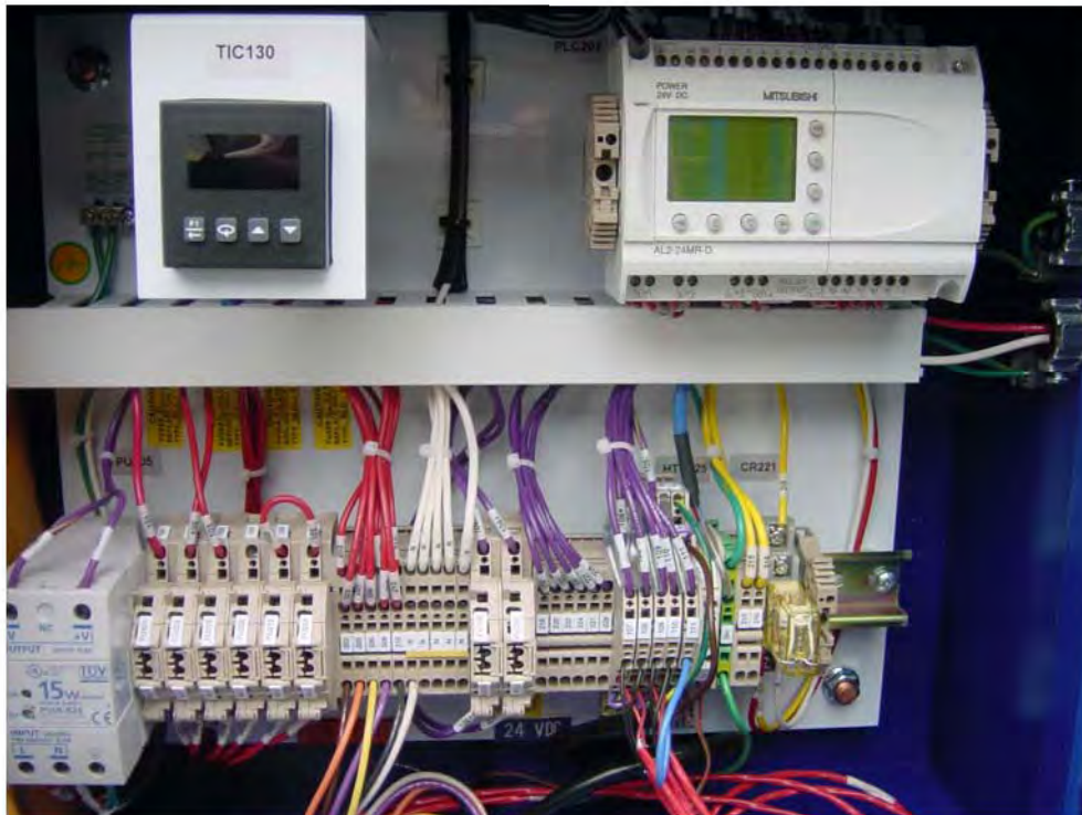
Figure 8 - Trifecta X-Series Control Box (open)
