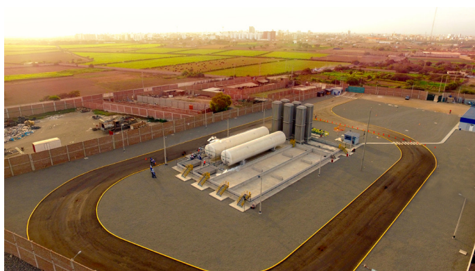
Figure 2. A series of small-scale LNG regasification facilities in Peru store LNG and provide natural gas to homes and businesses that previously used oil-based and wood fuels for heating.
