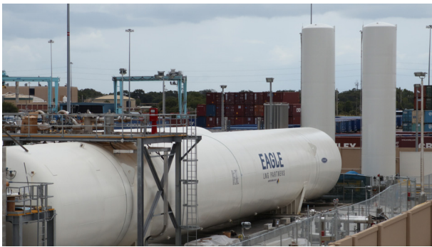
Figure 3. LNG bunkering terminal for fuelling ships in Jacksonville, Florida, US.
