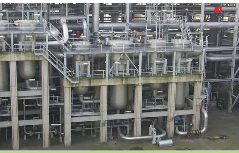
7 Hydrocracking Unit with VERTICAL LABLEX® Heat Exchangers - courtesy of SHELL PERNIS, NL
