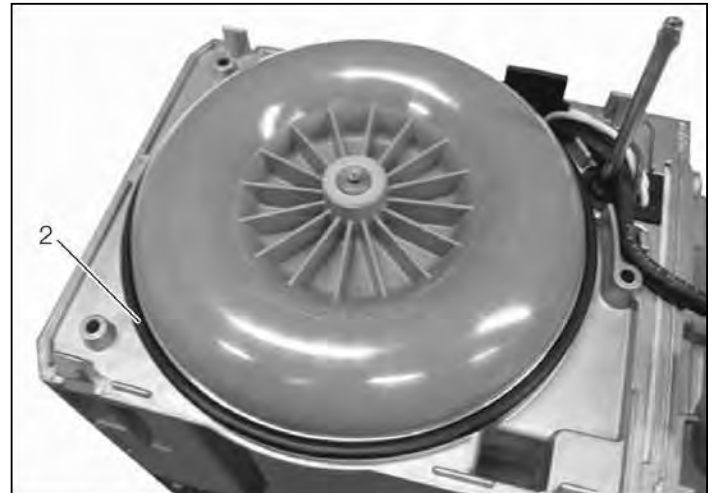
2 O-ring, positioned on the control box / blower unit.
