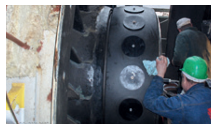
Elektrenai Power Plant, Lithuania, 2007. 150 MW(e) boiler. 1 and 2 stage fans with cast nickel alloy blades and rubber lined hubs and casings
