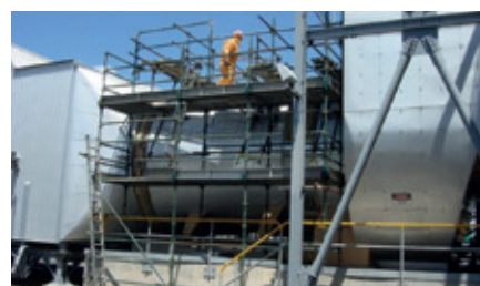
Kogan Creek Power Station, Australia 2006. 750 MW(e) boiler. 1 stage fan with aluminium blades
