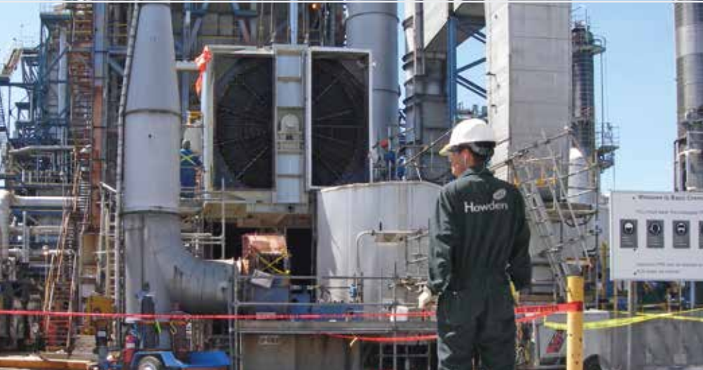
Figure 3: Installing the fully assembled unit
