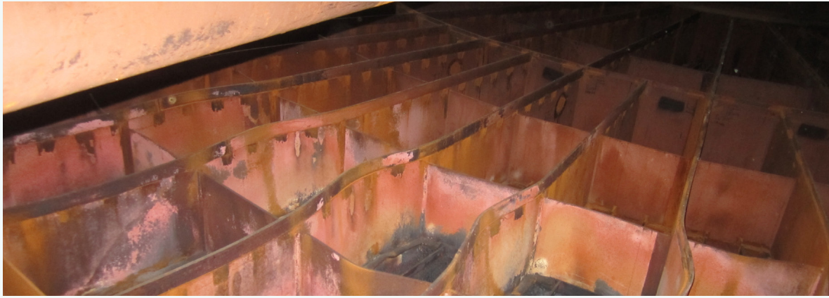
Basket damage caused by fire in an Air Preheater
