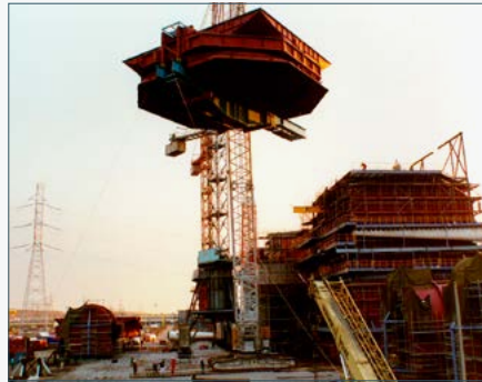
APH lift onto an FGD unit.
