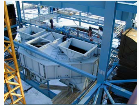
Quadsector APH installation
