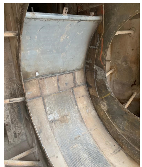
Figure 2: Cut-off section after wheel installation in perfect match.
