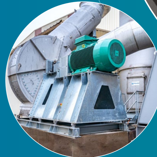
Insulation plant de-dusting fans
