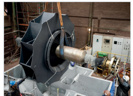
Installation of the new fan into its casing.
