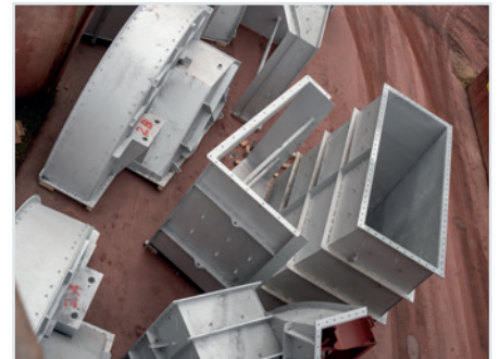
The new ducting awaiting installation.
