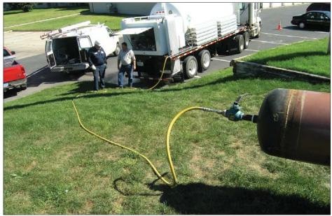
Pressure testing new underground pipelines is just one of many applications for the Liquid Tube Trailer HP<sup>2</sup>-2500
