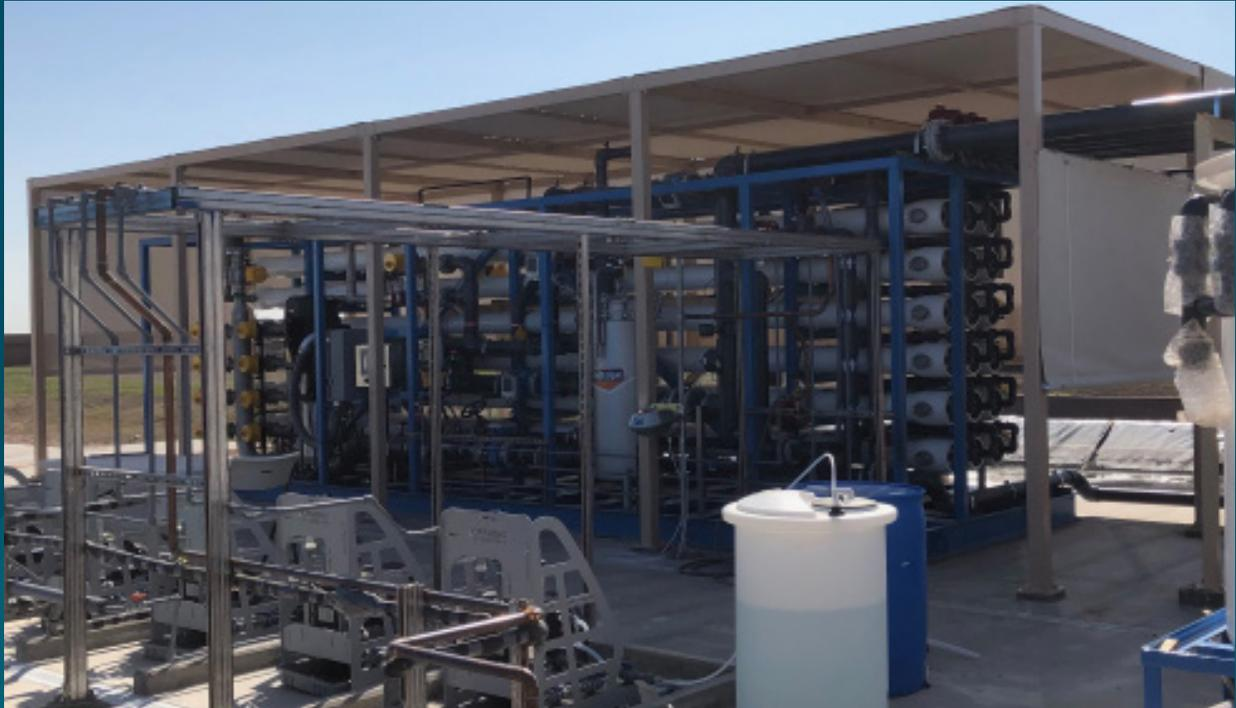
A 550 gallons per minute (feed) Flow Reversal RO system for removal of nitrate and TDS from groundwater located in Arizona, United States. The plant also includes pretreatment for removal of iron and manganese.
