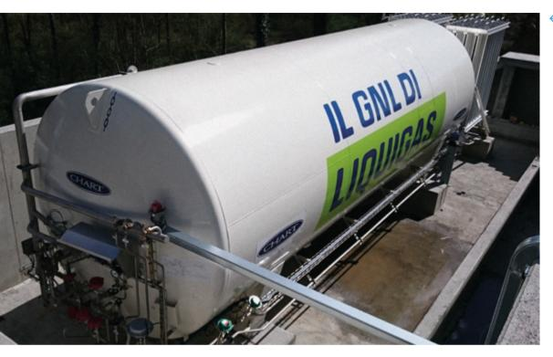
← Chart regasification plants store and re-vaporize LNG providing power plants or industrial users not connected to the pipeline grid with natural gas. Regasification plants can be configured for any demand requirement and comprise one or more vertical or horizontal storage tanks. They are typically supplied skid mounted to reduce project cost and complexity and facilitate easier transport and installation.
