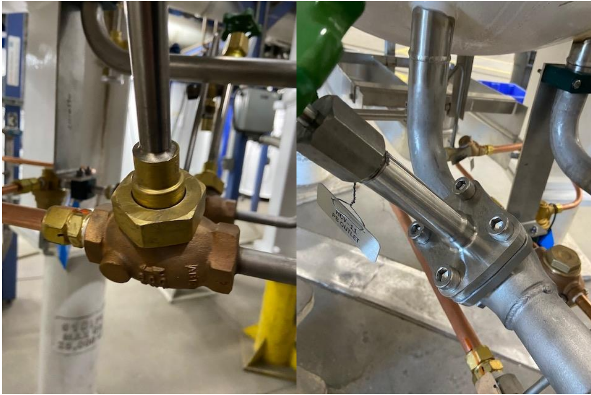
Figure 1. (Left) Current REGO BK Valve (Right) New REGO SK Valve
