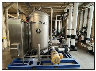
Control of existing diffusers had been achieved by manual adjustment of the CO<sub>2</sub> pound per hour (pph) delivery rate, requiring plant operators to constantly monitor pH in the recarbonation basins and adjust diffuser delivery rates accordingly. With pilot installed, operators could now know if the pH was right, on the spot, and maintain a set point. Benefit continues with permanent unit.
