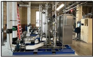
$\text{CO}_2$  had previously been added through round-plate diffusers to form bubbles that were hopefully small, but sometimes reached golf ball size. The piloted alternative method, and its permanent replacement, combines a side stream of water with carbon dioxide gas, in a pressurized saturation tank containing a gas head space, that is designed to create conditions ideal for dissolving carbon dioxide.
