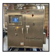
2013 pilot proprietary CO<sub>2</sub> dissolution and injection system had delivered typical CO<sub>2</sub> dose of 15 mg/L, while treating an average flow of 30 MGD (113,562 m<sup>3</sup>/day), and a range of 25-54 MGD (94,635-to-204,412 m<sup>3</sup>/day). Reduction in CO<sub>2</sub> delivery rate vs. diffusers was 21% to 57%, av. 40%, for projected annual savings in 2013 CO<sub>2</sub> cost and 2013 dollars of \$48,800 @ target pH 9.8, and \$124,000 @ target pH 8.5.
