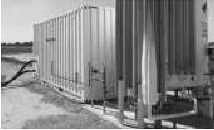
Figure 1: Drawing from a vertical, liquid oxygen tank, a containerized SDOX® unit oxygenates the wastewater in-pipe as it flows from the facility’s anaerobic lagoons before being pumped at a lift-station into the City’s collection system and eventual wastewater treatment plant. By maintaining an aerobic environment, the SDOX® unit mitigates odor and corrosion within the City’s collection systems while reducing the Company’s annual chemical treatment costs by an estimated $3.6 million.
