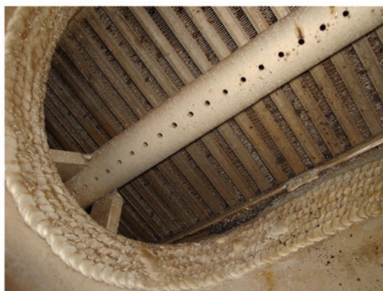
Figure 8. Fouling in header/nozzle.
