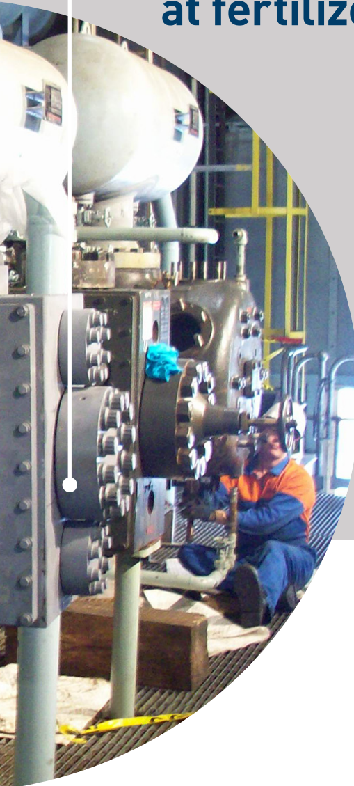
The new cylinder (near) featured thicker and stronger valve port walls, but that required redesigned valves to fit the smaller openings.
