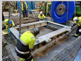
Base Plate installation
