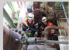
Bearing & Seal inspection & coupling replacement
