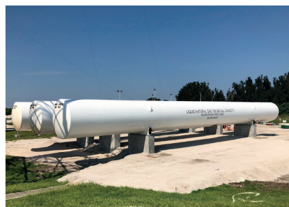
© Chart | (left) LNG Bullet Storage Tanks 3 x 100,000 gallon capacity; Multiple storage units with interconnecting VJ piping manifolds
