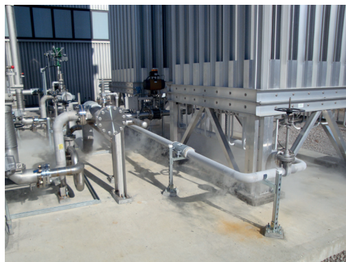
© Chart | Liquid nitrogen high pressure tank supply system at a space environment simulation chamber
