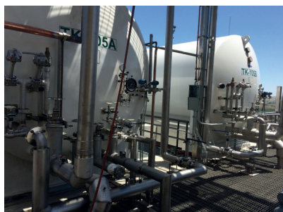
© Chart | (left) LNG Bullet Storage Tanks 3 x 100,000 gallon capacity; Multiple storage units with interconnecting VJ piping manifolds
