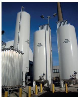
© Chart | Liquid nitrogen high pressure tank supply system at a space environment simulation chamber
