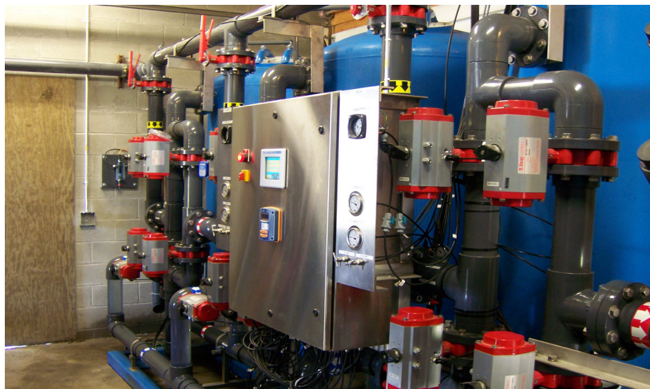
Each 48-inch diameter vessel contains 37 cubic feet of AdEdge's AD26 oxidation/filtration media.
