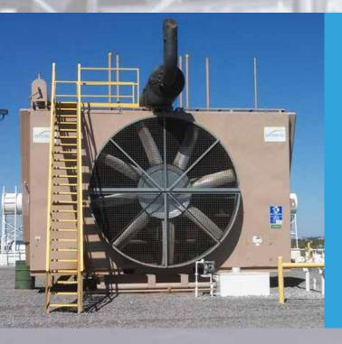
The Air-X-Changers Model EH is the world's most popular engine driven cooler.
