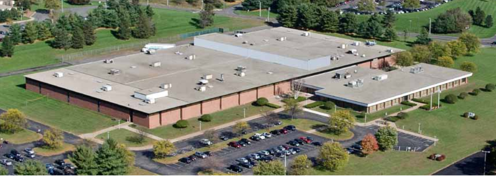
Spencer Corporate Headquarters and Manufacturing Plant, Windsor, CT USA
