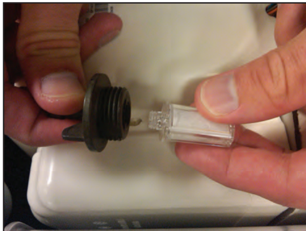
Figure 25 Installing the new HEPA Filter.
