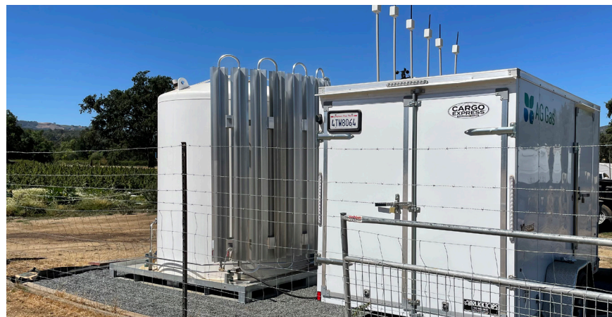
Perma-Max™ 12,000 VHP MicroBulk Storage System providing CO 2 for enrichment at a cannabis farm.
