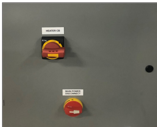
Figure 21 - High Voltage Panel for TBC (Exterior)
