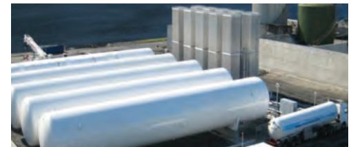
Mosjoen, Norway. Bunkering Station. 5 x 683m 3 tanks, pumps, and ambient air vaporizers.
