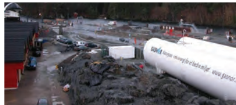
Halhjem, Norway Bunkering Station. 2 x 500m 3 tanks, pump and jetty module.
