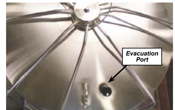
Photo 3 - Vacuum Evacuation Port with Cover
