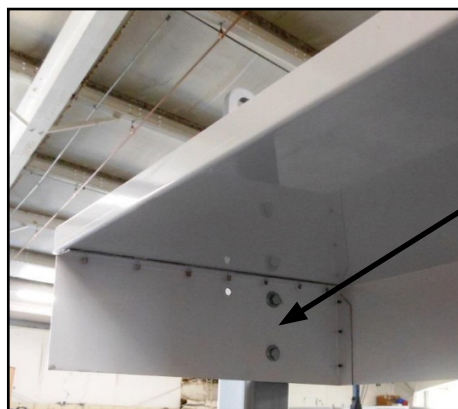
Figure 4 - Replacing bolts on awning
