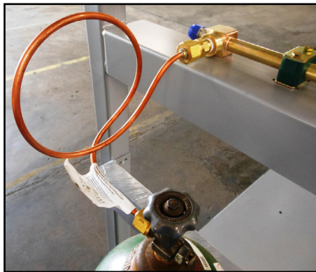
Figure 13 - Pigtail connections
