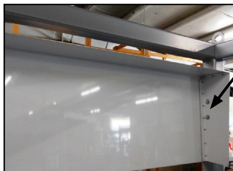
Figure 3 - Removing bolts on awning
