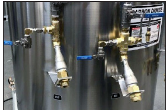
Figure 4 - Vapor Balance and Liquid Fill
