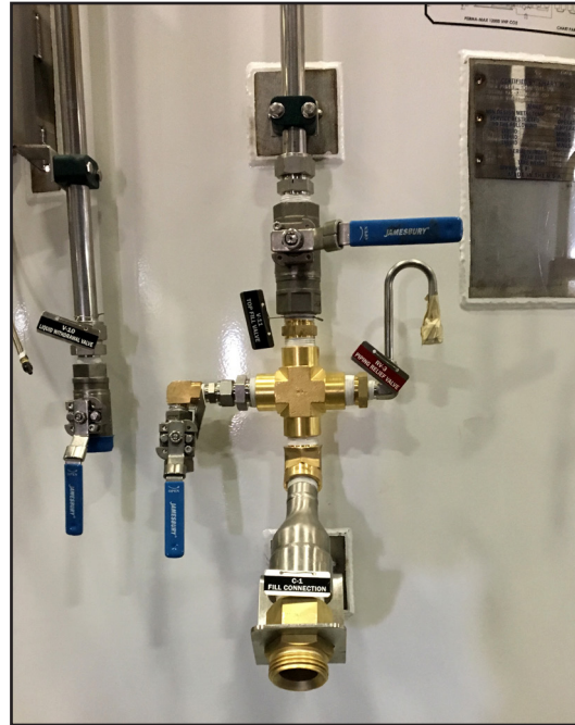
Figure 26 - Fill Valve (Shown with 1 1/2 CGA Bulk Fill Connection)
