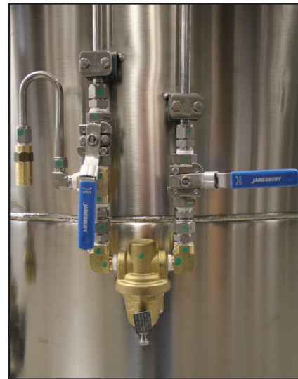
Figure 7 - Economizer Regulator with Isolation Valves
