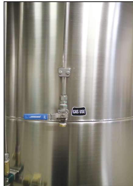
Figure 9 - Gas Use ball valve
