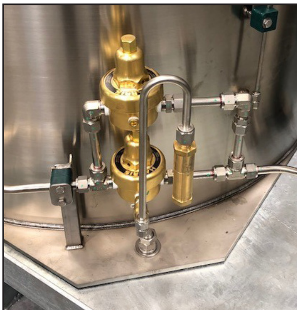
Figure 16 - Dual PB regulators
