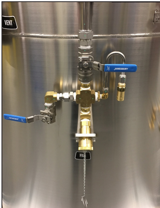
Figure 2 - Fill Line with Snap-Tite connection
