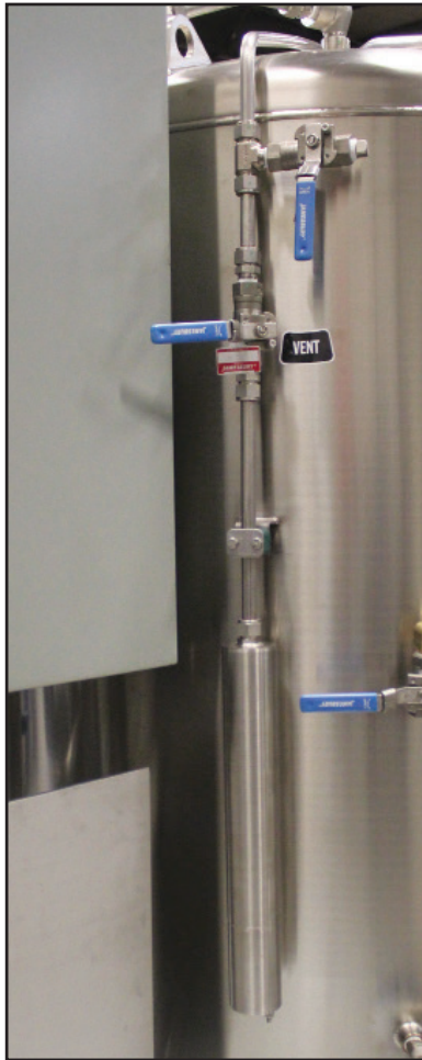
Figure 21 - Muffer on vent/full trycock plumbing circuit
