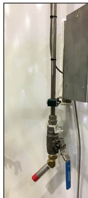
Figure 34 - Vent Valve/Full Trycock (V-4)
