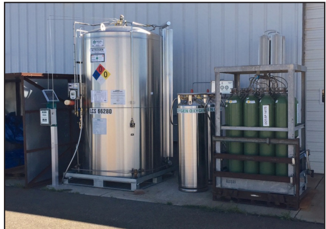
Figure 25 - Perma-Max 3300HP with external pressure build vaporizer
