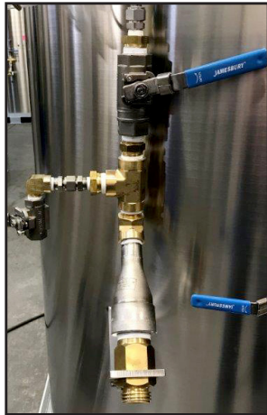
Figure 35 - Vapor Balance Kit
