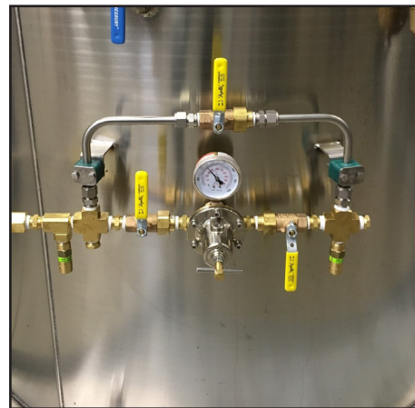
Figure 9A - Regulating manifold
