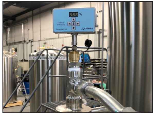
Figure 22 - C-Stic Liquid Level Gauge
