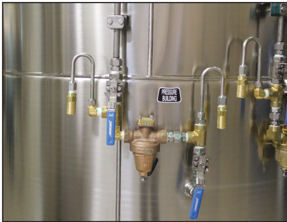
Figure 5 - PB Regulator with Isolation Valves
