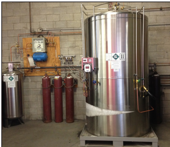
Figure 27 - Indoor Installation of a Perma-Max 3300HP tank
