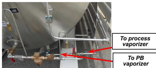
Photo 2 - Flow goes through the single PB regulator and splits to each vaporizer.
