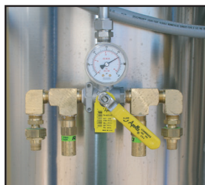
Dual Relief Valve Assembly
