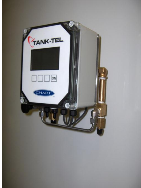
Figure 3.2.1-2: Tank-Tel III Gauge Assembly mounted onto tank.
