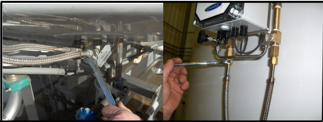
Figure 3.1.2-2: Tighten 0.313"OD x 0.035" WALL (P/N 11680638) ends with 11/16" Wrench.
