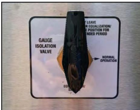
Figure 21 - Valve in "Equalization/Service" position
