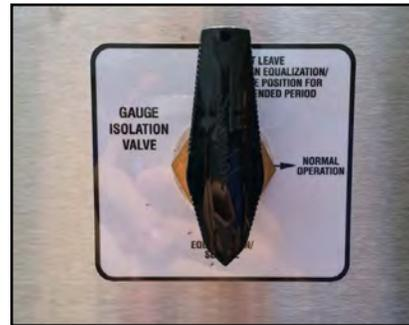
**Figure 2 - 5-way valve in the Equalization/Service position**
