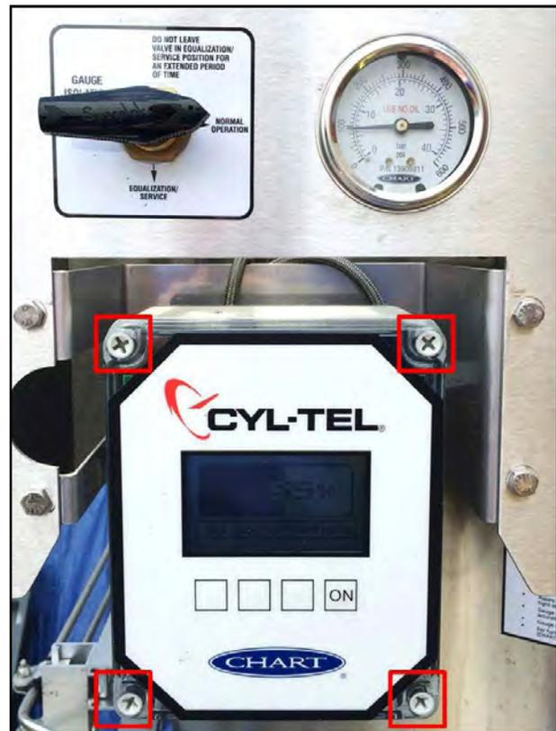
**Figure 6 - Red boxes indicate the four plastic screws that need to be removed**
