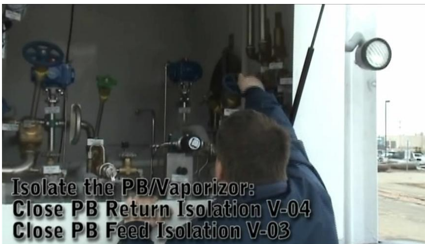
Figure 53 - close PB Return Isolation V-04
