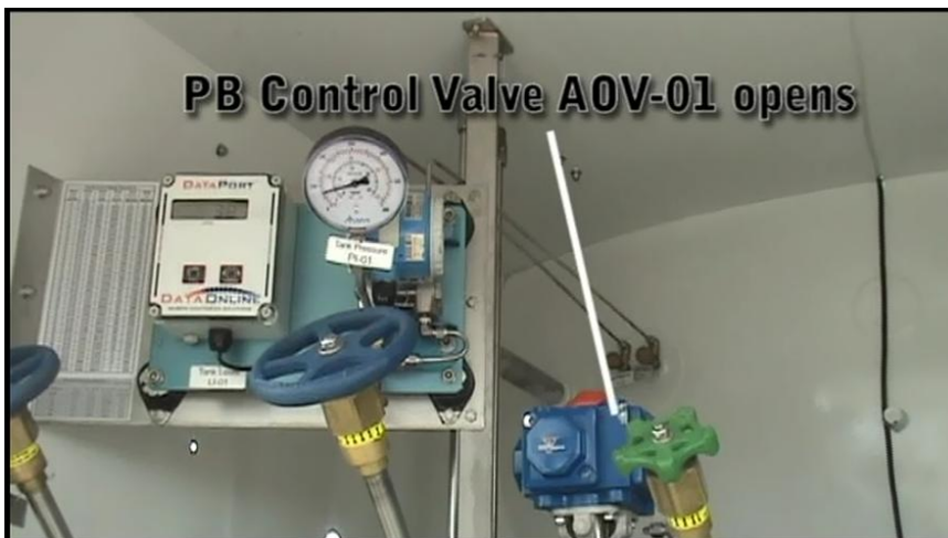
Figure 19 - PB Control Valve AOV-01 opens
