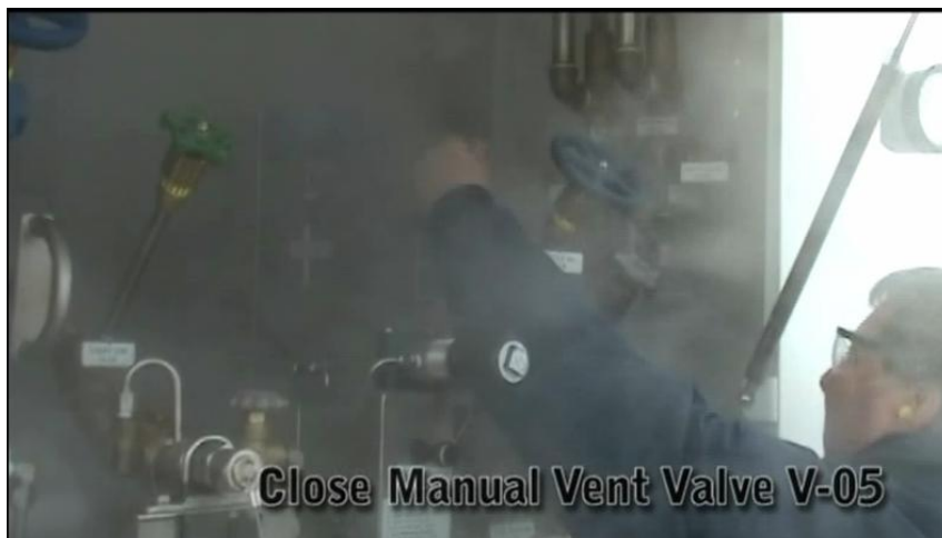
Figure 27 - Close Manual Vent Valve V-05
