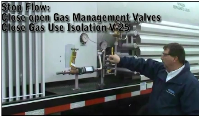
Figure 43 – close open gas management valve
