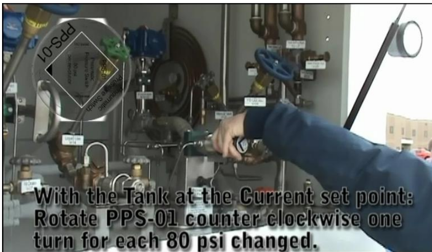
Figure 24 - Rotate PPS-01 counter clockwise for each 80 psi changed
