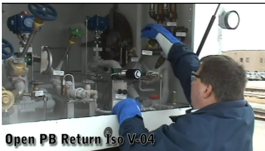
Figure 61 - open PB Return Iso V-04
