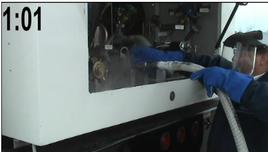
Figure 64 – connect inlet side of hose
