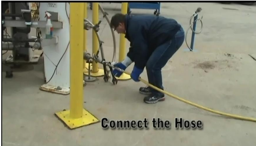
Figure 32 - connect the hose
