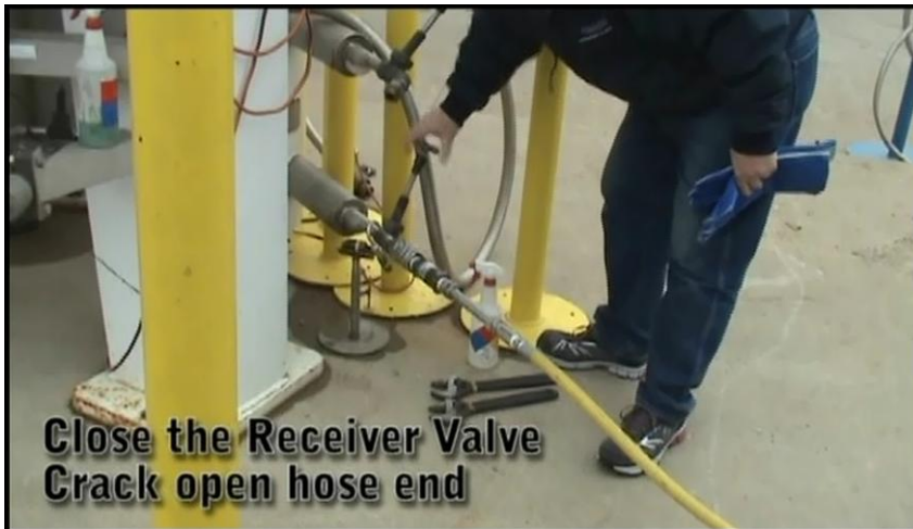
Figure 46 - crack open hose end
