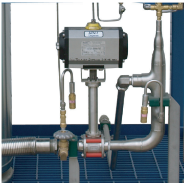
Automatic Fill and Safety Shut-Down Valve
