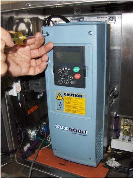
Remove the front cover of the Variable Frequency Drive by loosening the four Phillips head screws, located near the corners as shown.
