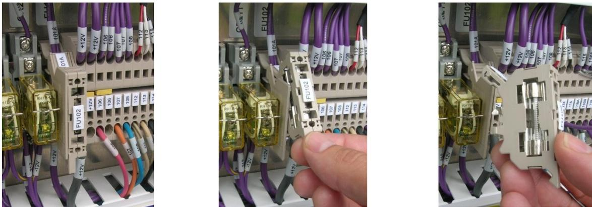
Fuse FU102 protects the 12VDC circuits and components downstream of the 12VDC terminal block from over voltage conditions. The fuse can be accessed by lifting up on the tab and giving a slight twist to the fuse holder as shown in figure XX. The fuse used for the system is a BUSS MDL-10. For more details of the 12 VDC system, see Section 4 of this manual for complete electrical schematics.
