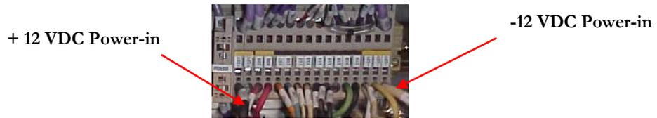
6. Is the 12 VDC Fuse FU102 blown? Open Fuse access and ohms check the fuse.
