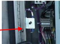
5. Is there 12 VDC Power to Terminal Strip 1? Use a Voltmeter to check the 12 VDC Power-in to Terminal Strip 1.
