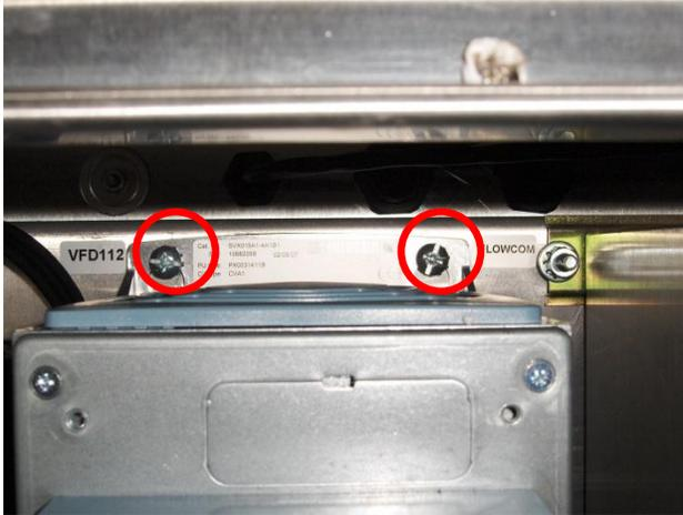
Loosen the four VFD mounting bolts located at the four corners of the VFD far enough to allow it to be lifted out of its mounting position. (Upper mounting bolts shown)
