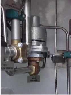
The Hose Drain Solenoid, located behind the Low Flow dispense valve, is a Normally Open Solenoid. This allows a path for product left in the dispense hose following a delivery, to return to the sump. This solenoid becomes active and closes off the path in unison with the dispense valve opening when dispensing product. The Hose Drain Solenoid is part of the 12 Volt DC system and receives a power signal from the FlowcomS8. No maintenance is required for this part.
