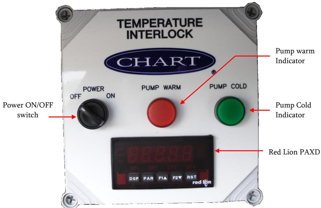
When the temperature will not drop any further, this Value is entered into the Red Lion Programming. The total time of the cool down is also recorded. This time, plus an additional 5 minute delay is entered into the Red Lion Programming to ensure proper and adequate cool down before the GREEN "PUMP COLD" light illuminates. Once these conditions have been met, the pump can be operated.
