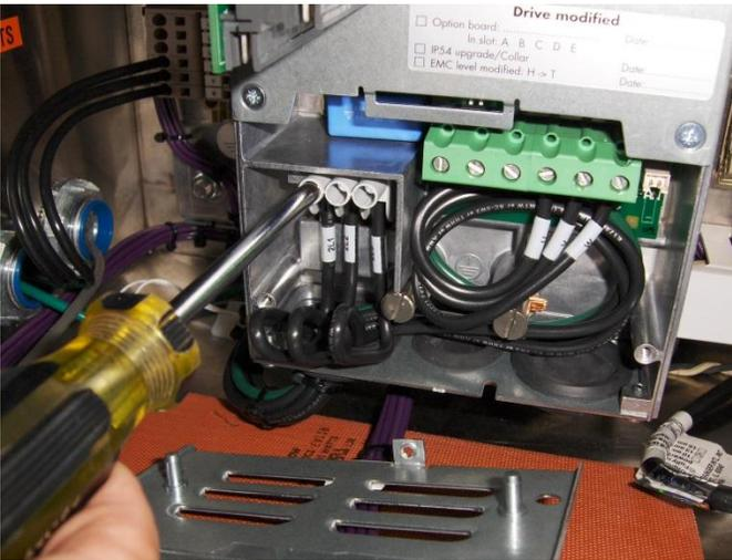
Remove the three incoming 480 VAC wires (2L1,2L2,2L3), and the three outgoing 480 VAC wires (U,V,W), as shown.
