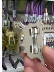
7. Is there 12 VDC Power to the Low Voltage Junction Box? Use a Voltmeter to check the 12 VDC Power to the Low Voltage Junction Box.
