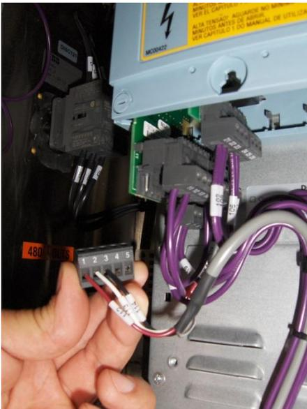
With the front cover removed unplug the 12 Volt wiring as shown, noting the position of each plug for installation into the replacement VFD. The numbers are aligned 1-26,
