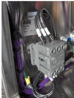
When the 480 Disconnect switch is turned to the “ON” position, the 480VAC from the Alternator is supplied to the 480VAC Contact Block in the control cabinet. Will this switch in the “OFF” position, it is not possible to power the VFD or the Pump.
