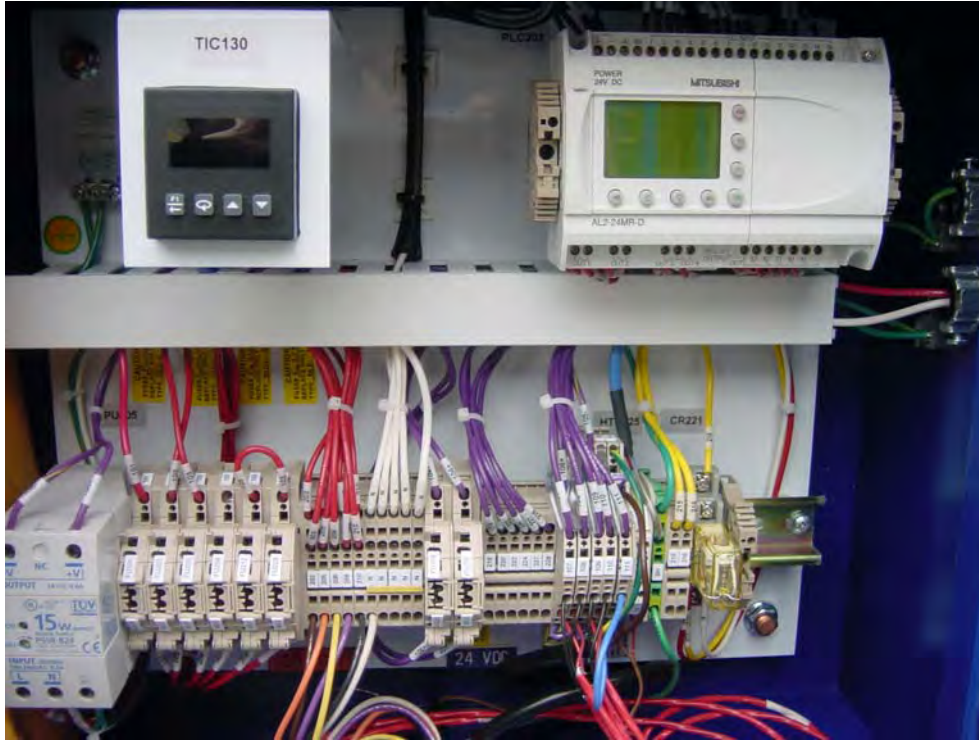
Figure 9 - Trifecta X-Series Control Box (open)
