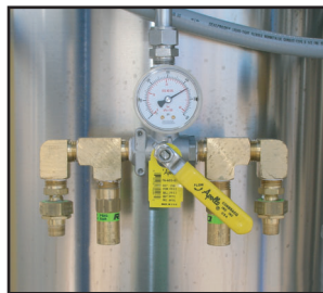
Dual Relief Valve Assembly
