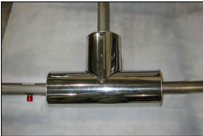
12. After completion, T-joint should look like this.
