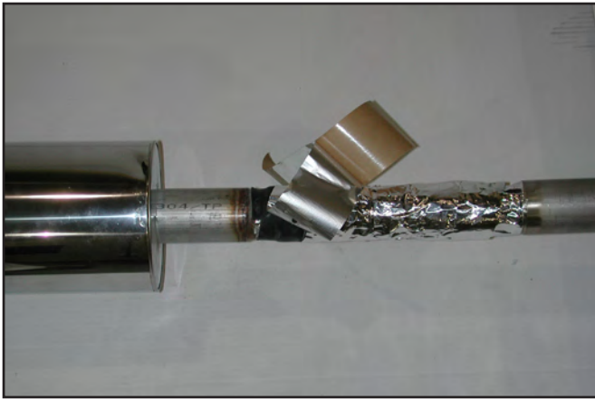
7. Wrap a layer of aluminum foil tape over section A over the foam insulation.
