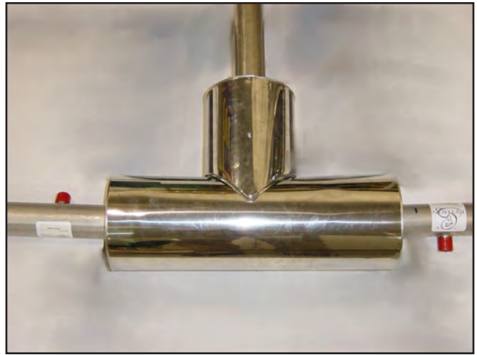
10. Slide small T-joint cover over aluminum tape and attach it to longer T-joint cover. • Put end on • Line up holes • Put screws in
