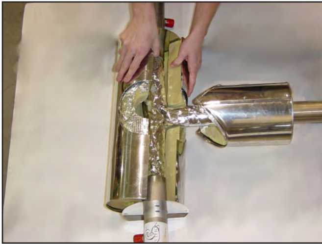
8. Put longer T-joint section (metal cover and insulation) over aluminum foil tape by sliding it around pipe.
