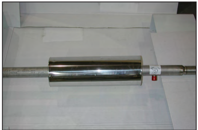
11. Completed joint installation should look like this.
