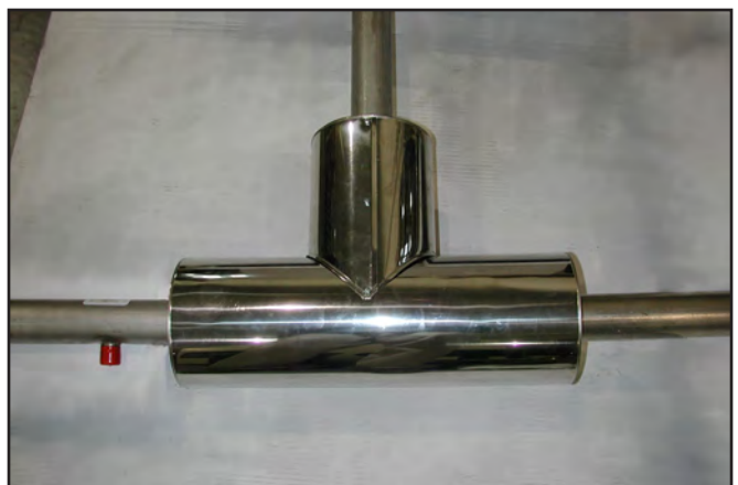
12. After completion, T-joint should look like this.
