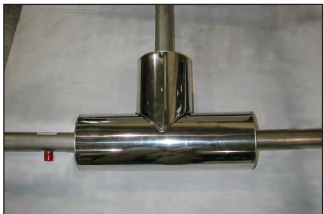
12. After completion, T-joint should look like this.
