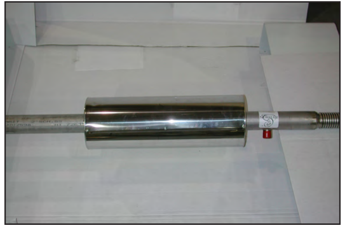
9. Slide or place cover over aluminum tape and insulation to the marks on pipe (made in step 1) or until cover is centered over joint.
