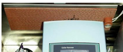
Control Panel Heater
