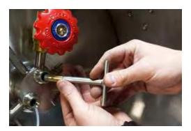
Clean/replace fittings, tape pipe threads per VT-0030, install new Flaretite seals on flared fittings, and reinstall plumbing. Refuel tank and check connections for leaks before returning unit to service.
