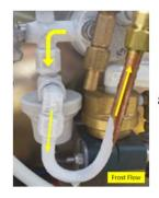
Note: After several minutes of operation frost will begin appearing throughout the plumbing due to radiant cooling and liquid settling to low points in the plumbing.
