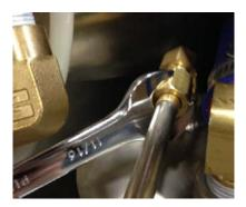
24. Using 11/16" combination wrench, tighten the nut of compression fitting end on the Excess Flow Valve.
