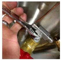
16. Remove any remaining thread sealant tape from the shut off valve female pipe threads using a wire tube brush. Open the valve for a few seconds to purge out any remaining debris then close it.
